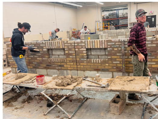
1st Year Correspondence Brick Apprentices Brock Lizotte and Darrin Aleckson working together to build a brick and block window wall project.
