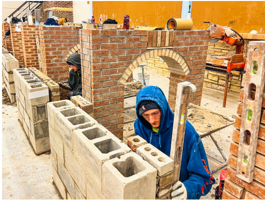
3rd Year PCC Apprentices Alex and Zachary Johnson building a brick and block project featuring a soldier detail.
